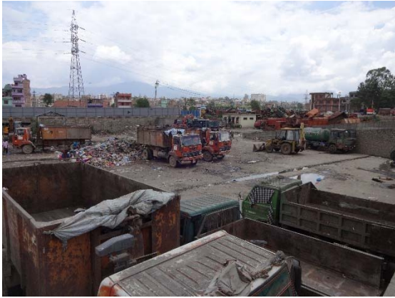
Figure 4.40 Existing solid waste management facility in Teku
