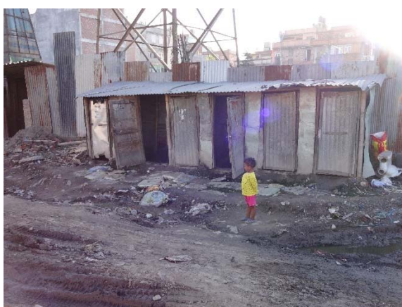
Figure 4.12 Communal toilets in Balkhu
