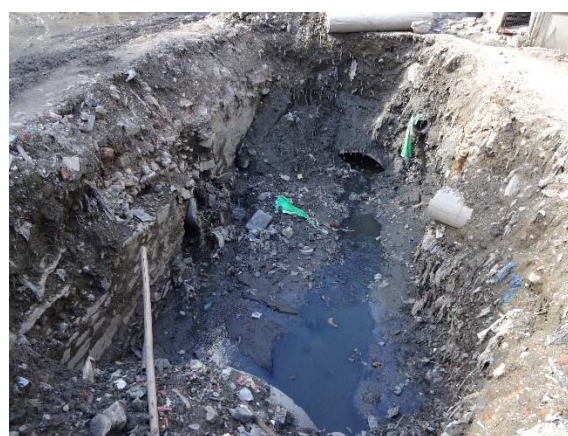
Figure 4.13 Excavated toilet discharge pipes and standing blackwater in excavations
