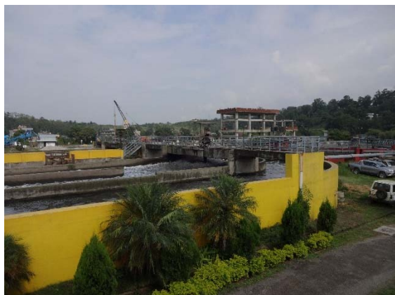
Figure 4.34 Existing WWTP at Guheshowri Source: (R Dewhurst 2017)
