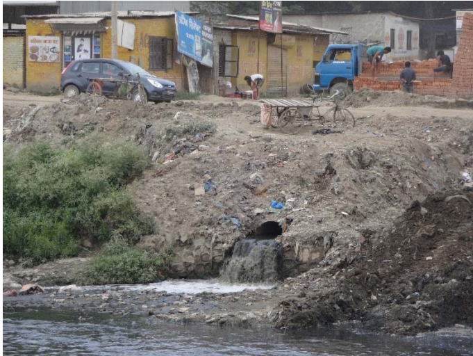
Figure 4.36 Untreated sewer discharge direct to the Bagmati river near Balkhu
