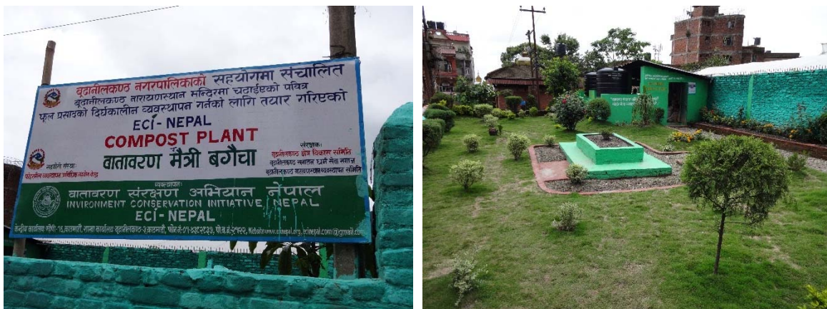
Figure 4.42 Compost plant near the Budhanilkantha Temple north of Kathmandu
