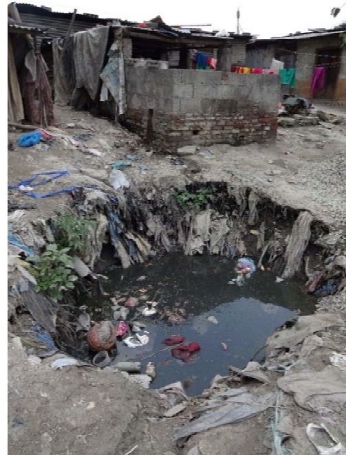
Figure 4.33 Blackwater accumulation adjacent to damaged toilet discharge
