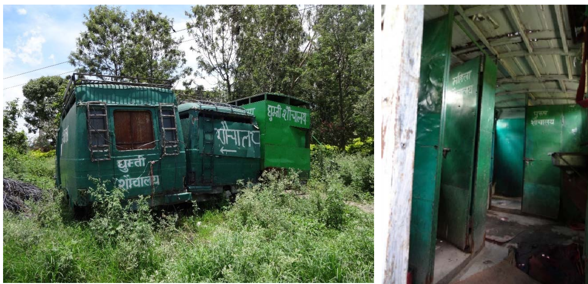
Figure 4.47 Abandoned mobile toilet units at KMC in Teku
