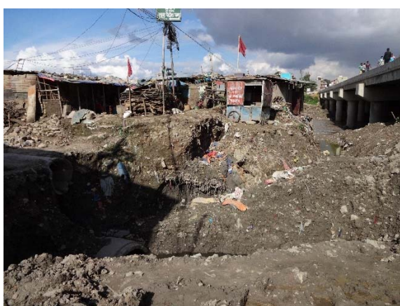
Figure 4.10 Access to Balkhu from the ring road
